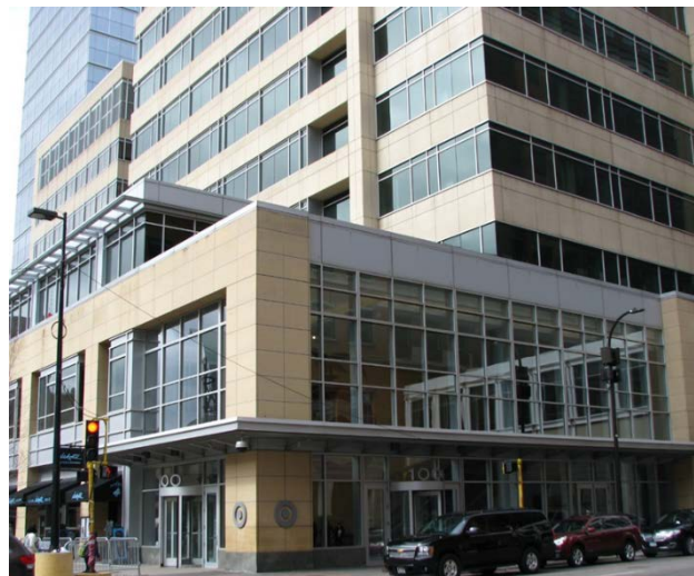
Target Headquarters, Minneapolis, MN. ENERGY STAR certified in 2016.
